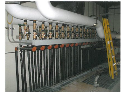
3 The loops are filled with fluid, which absorbs heat from the earth.
