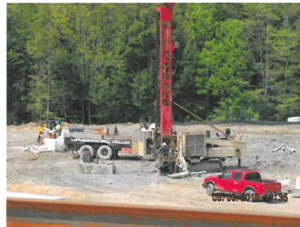
1 Fifty-nine bore holes were drilled to a depth of 400 feet.
